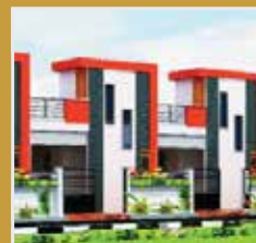
ASHTA MANGALAA VILLAS @ Ponneri
